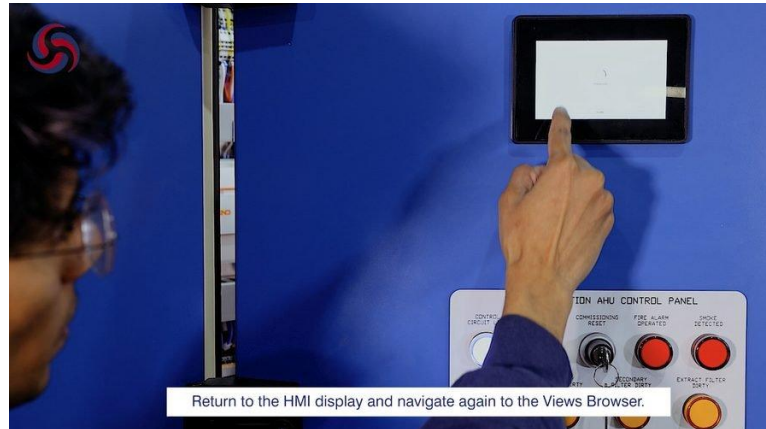
Figure 9. Returning to the HMI display and navigating again to the Views Browser to verify restored values.
