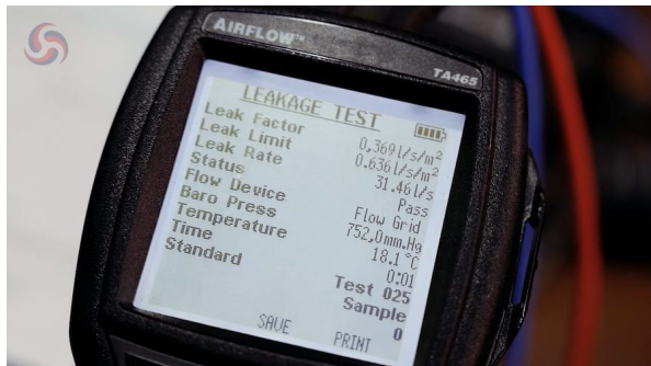
Figure 12. AIRFLOW PANDA TA465 leakage test display — Leak Factor, Leak Limit, Leak Rate, Status: Pass.
