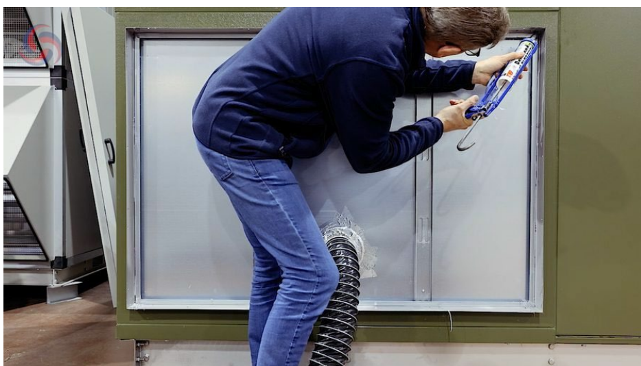
Figure 5. Sealing of AHU connections.
