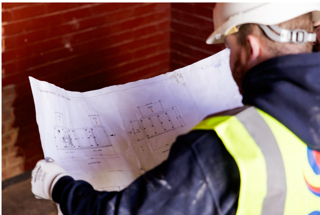
Figure 2. Site personnel in PPE reviewing the certified drawing. Confirm test pressure, leakage classification and sealed openings before pressurising the AHU.
