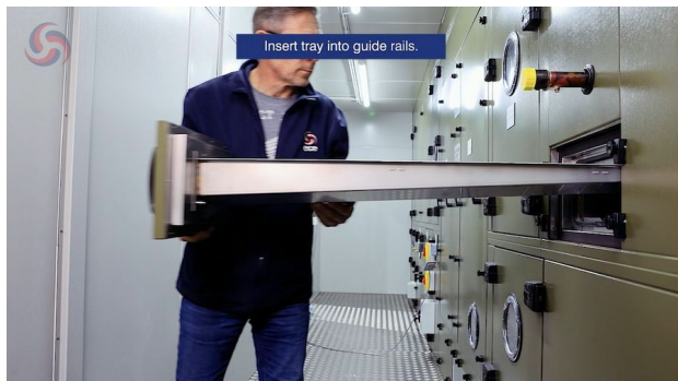
Figure 6. Sliding the cleaned drain tray fully back into the guide rails.
