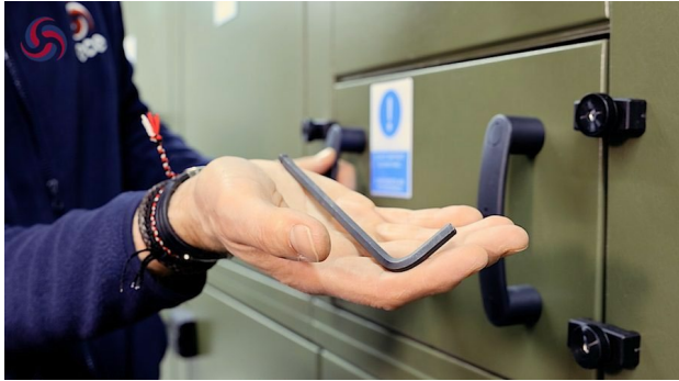
Figure 2. Identifying the retaining-panel fixings — Allen key or finger-tight fasteners may be used.
