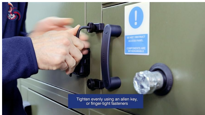
Figure 8. Tightening fasteners evenly with an Allen key or finger-tight fasteners. Do not overtighten.
