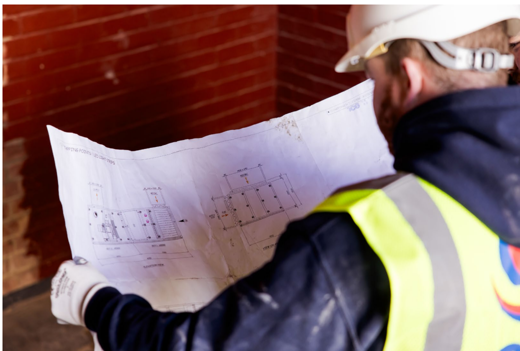
Figure 2. Site personnel in PPE reviewing the certified drawing. Confirm AHU identity and the project-specific drain/condensate arrangement before opening any access panel.
