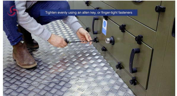
Figure 11. Tightening the fixings evenly using an Allen key or finger-tight fasteners.
