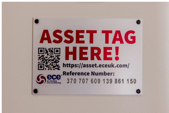
Figure 3. Asset Tag plate carrying the unique 18-digit reference number used to retrieve AHU technical information from the ECE Client Portal.
