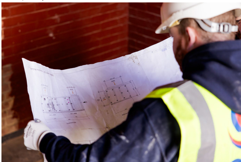
Figure 2. Site personnel in PPE reviewing the certified drawing. Confirm AHU identity and the project-specific drain/condensate arrangement before opening any access panel.
