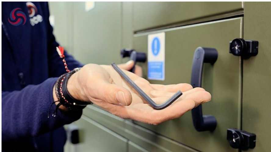
Figure 4. Identifying the fixing type — an Allen key is used here for the access panel bolts.
