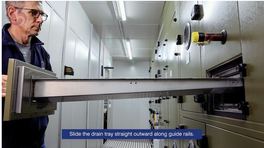
Figure 6. Sliding the stainless-steel drain tray straight outward along the guide rails.
