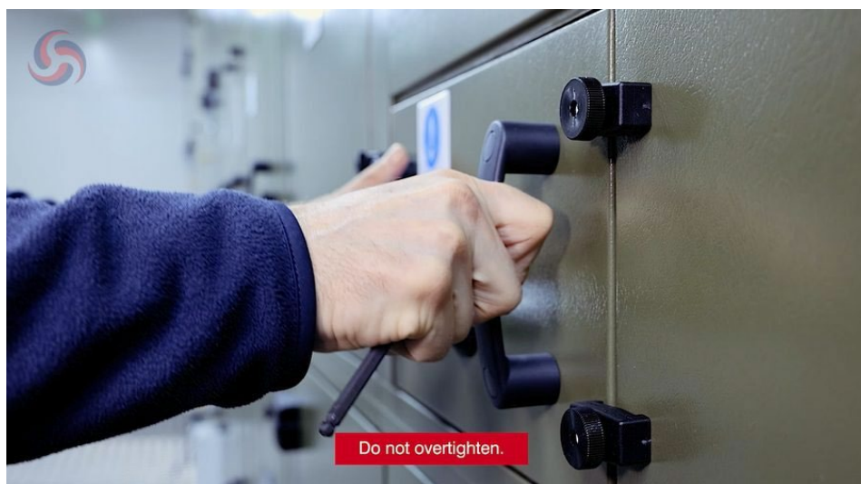
Figure 12. Do not overtighten — the panel must sit flush and maintain an air-tight seal.
