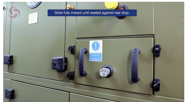
Figure 9. Tray slid fully inward until seated against the rear stop, level and square.
