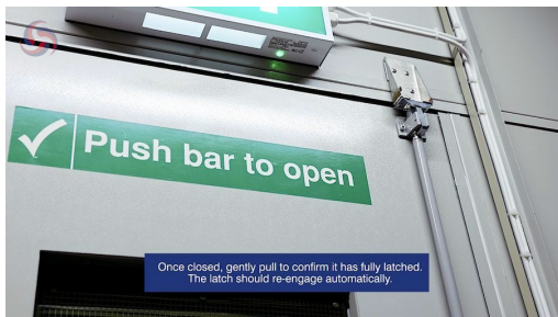
Figure 8. Confirm latch engagement: gently pull the closed door — the latch should re-engage automatically.
