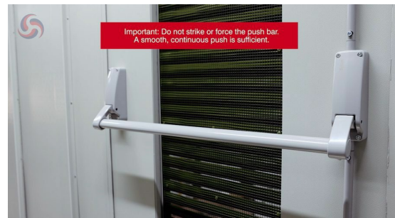
Figure 6. Do not strike or force the push bar — a smooth, continuous push is sufficient.
