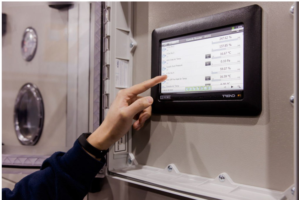
Figure 2. Typical HMI display fitted to ECE air handling units. Maintenance alarms are viewed and reset directly from this display.
