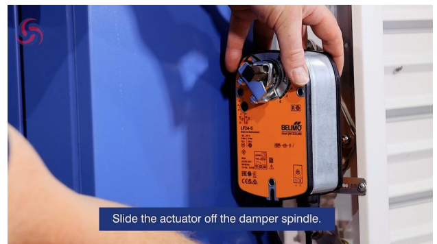
Figure 10. Sliding the actuator off the damper spindle once the clamp is released.
