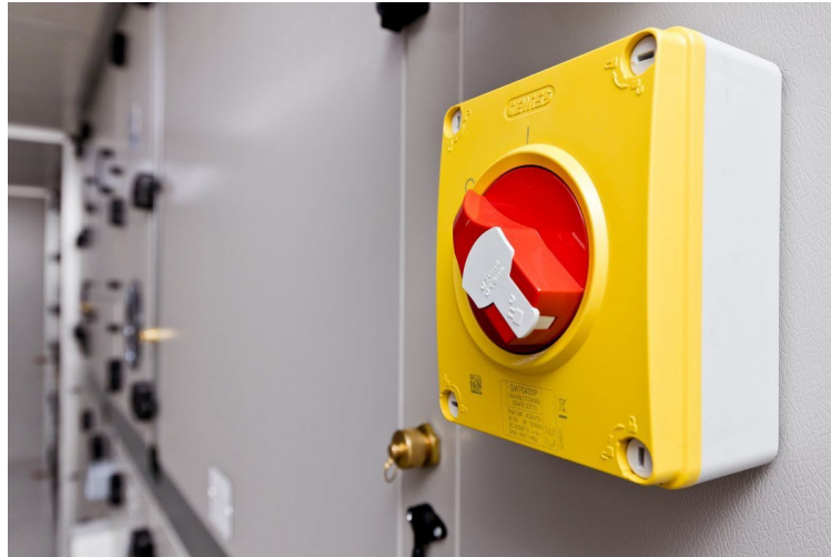
Figure 19. Verifying actuator status, control signal and damper feedback at the 5-inch HMI display.
