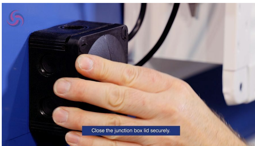
Figure 15. Closing the actuator junction box lid securely. Confirm no exposed conductors remain visible.
