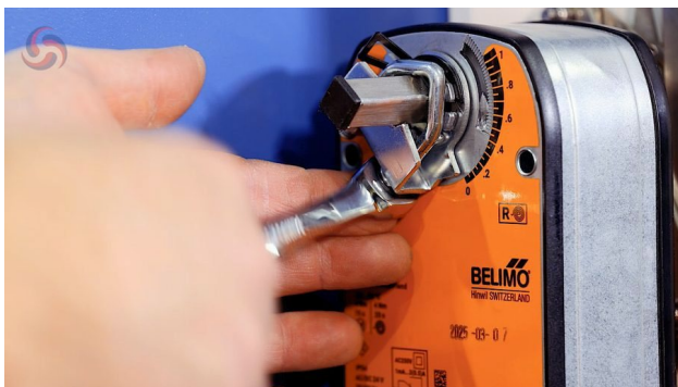
Figure 9. Releasing the actuator clamp from the damper spindle.
