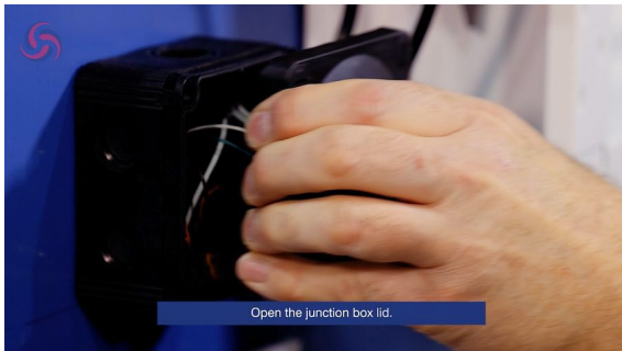
Figure 7. Opening the actuator junction box lid to access the terminal block.
