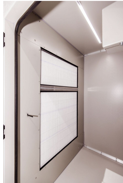
Figure 16. Alternative view of the filter section showing the tubing route from the tap-off point alongside the filter face.
