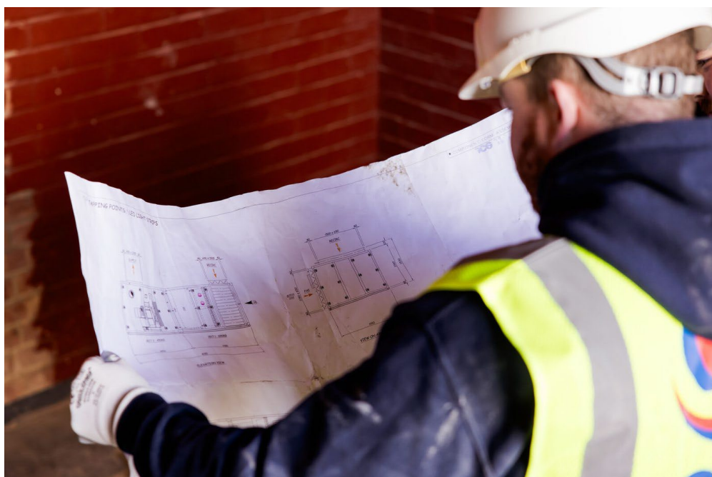
Figure 2. Site personnel reviewing the certified drawing for the AHU before commencing work on the Magnehelic gauge.
