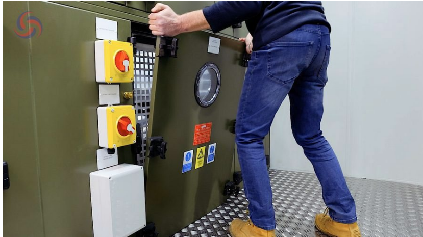
Figure 8. Lifting the door vertically from the frame.
