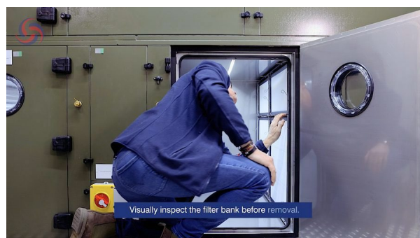
Figure 4. Visually inspecting the filter bank before removal.
