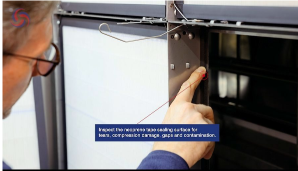
Figure 7. Inspecting the neoprene tape sealing surface for tears, compression damage, gaps and contamination.
