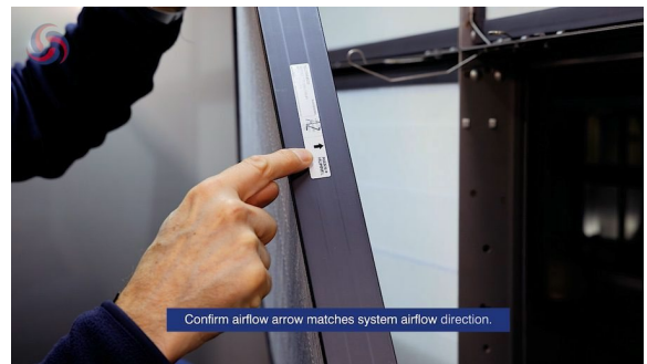
Figure 10. Confirming the airflow arrow on the new filter matches the system airflow direction.
