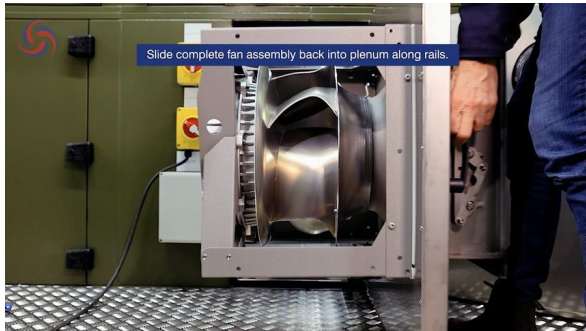
Figure 21. Sliding the complete fan assembly back into the plenum along the rails. Ensure the frame is fully seated.
