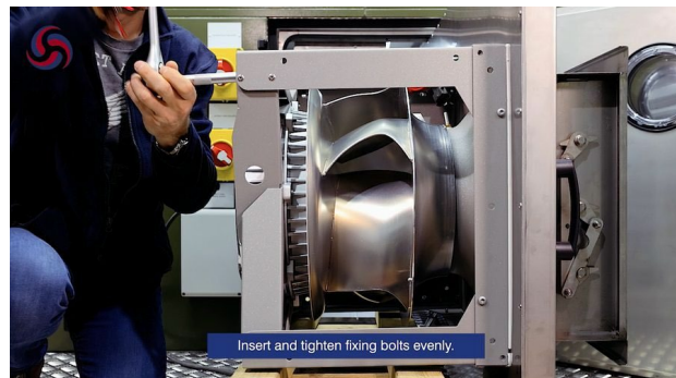
Figure 19. Inserting and tightening the fixing bolts evenly.
