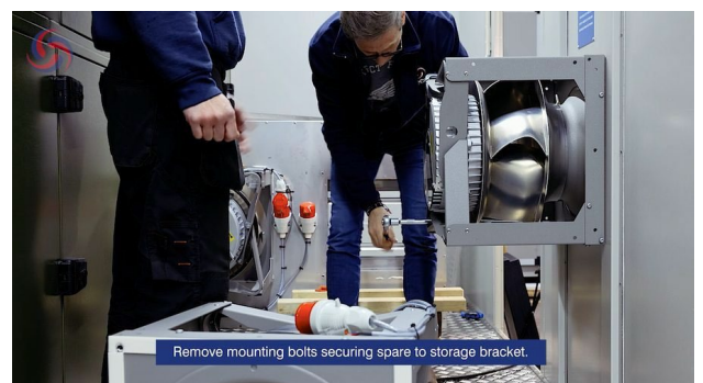
Figure 17. Removing the mounting bolts securing the spare fan to its storage bracket.
