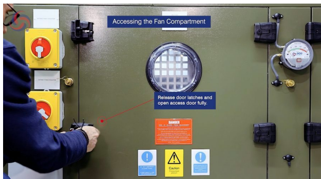
Figure 7. Releasing the door latches and opening the access door fully to reach the fan compartment.
