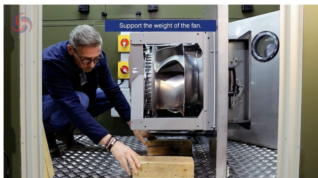
Figure 11. Supporting the weight of the fan after the assembly is slid outward along the EasyShift rails.
